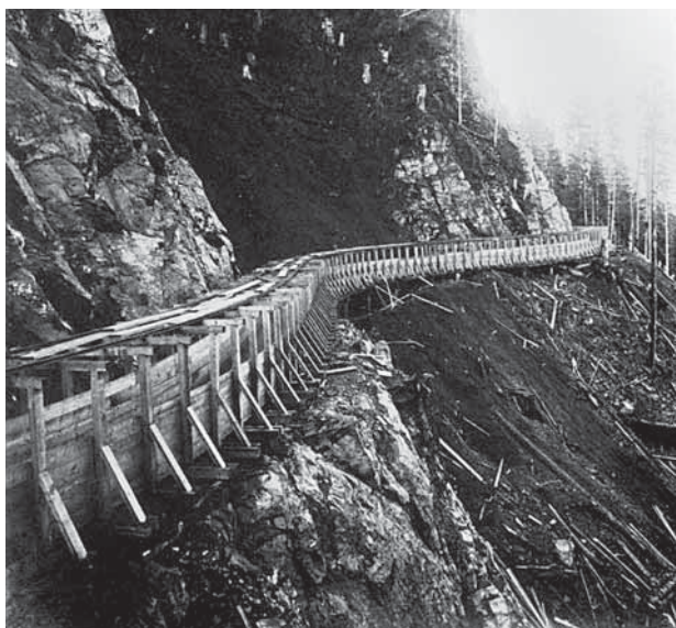
Flume construction through the canyon near Camp 4 of the Electron power station, December 31, 1903. Courtesy of the University of Washington libraries, Special Collections, Puget Power 206. From In The Shadow of the Mountain , by Lawrence D. Anderson.
