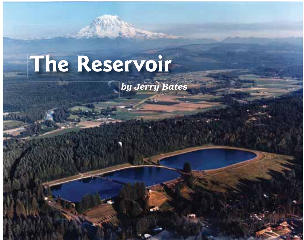
Tacoma Public Utilities McMillin Reservoir, part of our history
