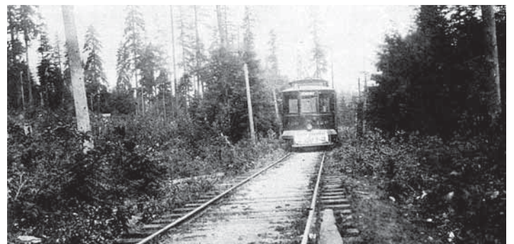
Thanks to member Dorothy Norris for this picture of the Old Line making its way up the Hill.
